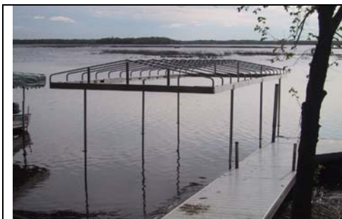
Six support posts hold the Sea-Legs Canopy Frame Top.
